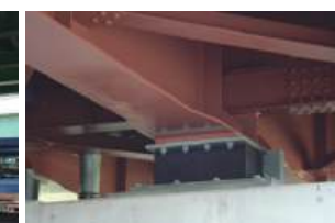
Bridge-Use Lead Rubber Bearing (LRB®)
